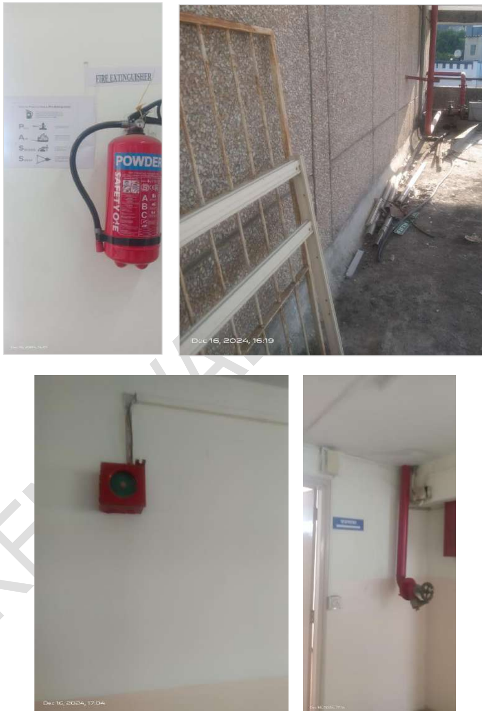
Plate 5: Fire and life safety measures undertaken
